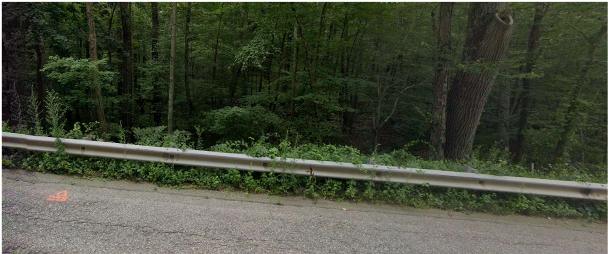
Example of grade behind the guardrail.
